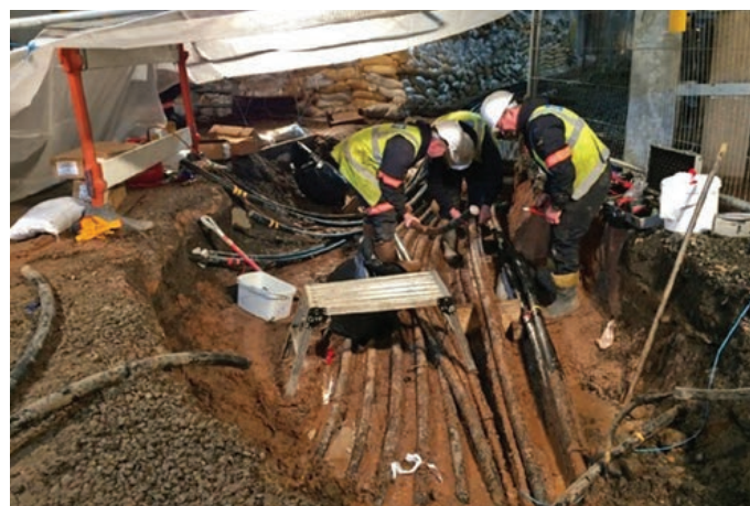
Figure 8: Laying high-voltage cables outside the substation (photo: courtesy of Electricity North West)
