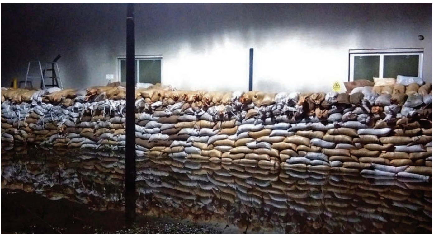
Figure 4: Sandbags at Lancaster substation (photo: courtesy of Electricity North West)
