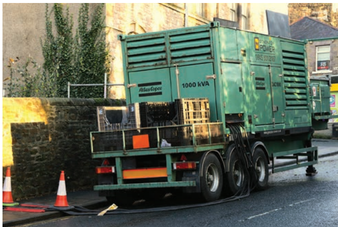
Figure 5: Generator in Lancaster, connected to local substation
