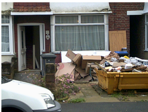
Fig. 3. Gutting the house.
