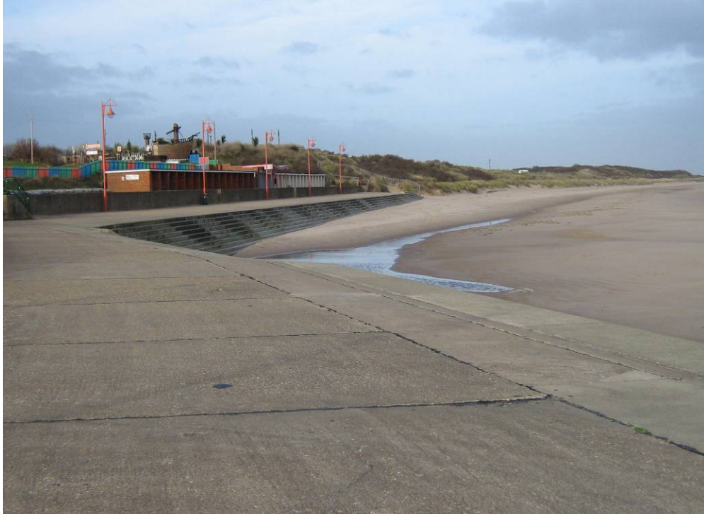
Plate 5.1: Looking north along the sea defences at Mablethorpe from 'Kids Adventure World'. NB. Three forms of defence are visible; the dune system, the nourished beach and the engineered concrete seawall.
